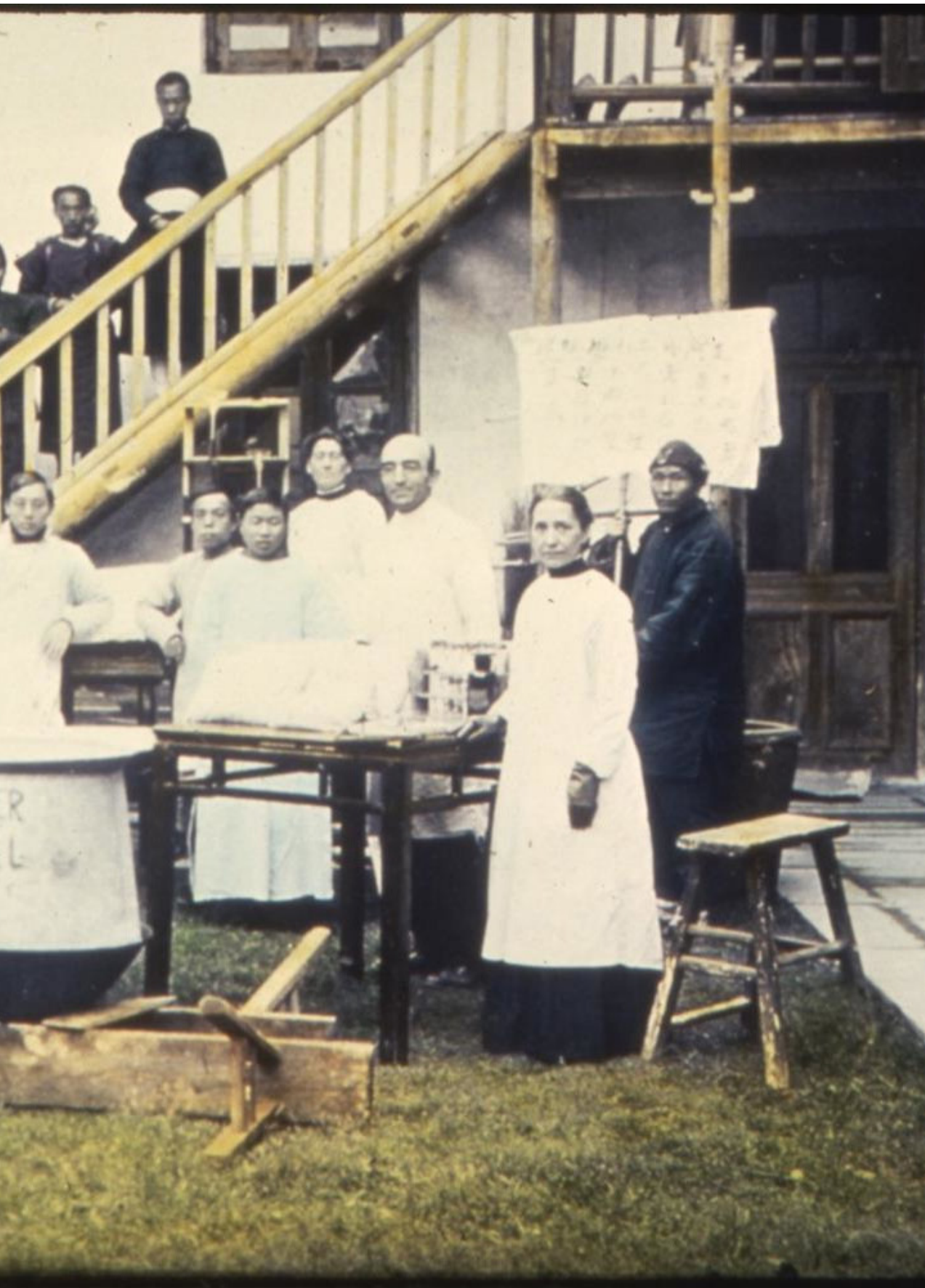
Hospital staff and volunteers with water distillation apparatus during cholera epidemic. A Chinese worker used two large woks to fashion the apparatus, in which 1.5 tons of sterile saline solution was made. (Jennie Logan is sixth from left; Dr. Logan is third from right). Changde, Hunan ca. 1912
